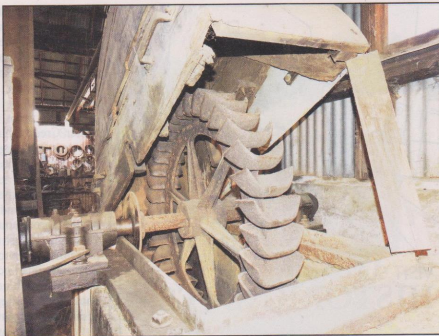
A water wheel that powered the Knight Foundry.
